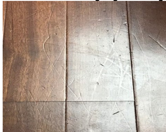
Dent & Impact (not scratches because finish is not abraded)
